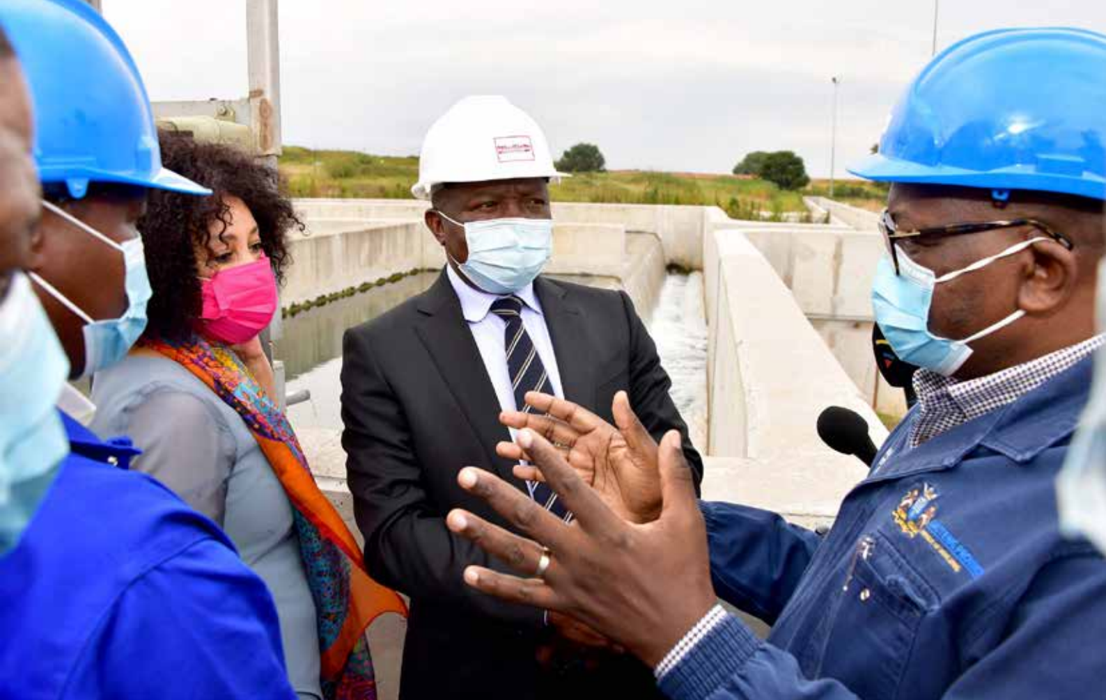
Deputy President David Mabuza undertakes a guided tour of the Sebokeng Waste Water Works during a visit to Emfuleni Local Municipality, Gauteng Province, March 2021
