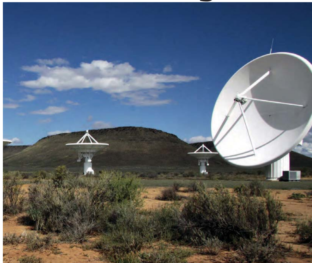
GROUND BREAKING: The construction site of the Square Kilometre Array telescope in the Karoo. As a great astronomy hub, South Africa is ready to host the telescope.
