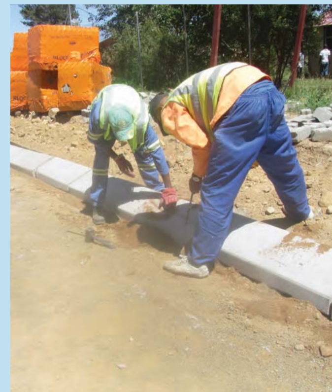
JOB CREATION: Construction workers busy building a road in Batho township.
