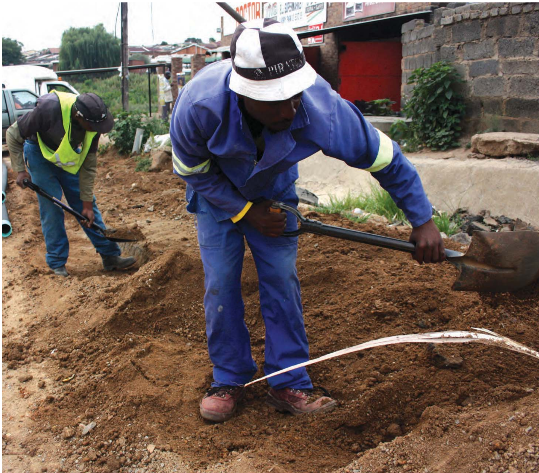
FOUNDATION FOR THE FUTURE: Construction workers in Ivory Park.
